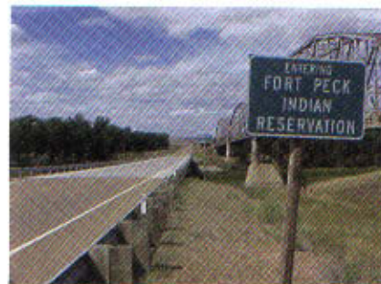
Sansaver grew up about a half mile from this site on land he inherited from his mother. Both the old and new bridge spans the Missouri River which is the southern boundary of the reservation.
