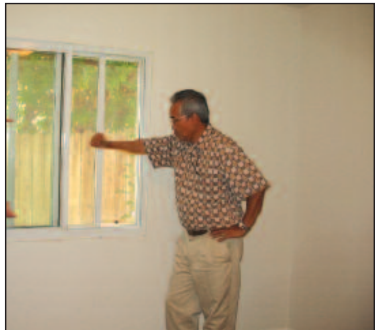
At a model home owned by the city, Ruben Cabalbag demonstrates how the customized double-paned windows prevent noise while maintaining egress regulations.
