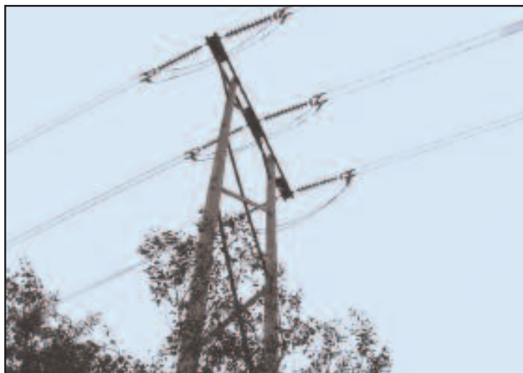
Telephone wires - Tree and vegetation encroachment in the ROW is a major issue for electrical utilities
