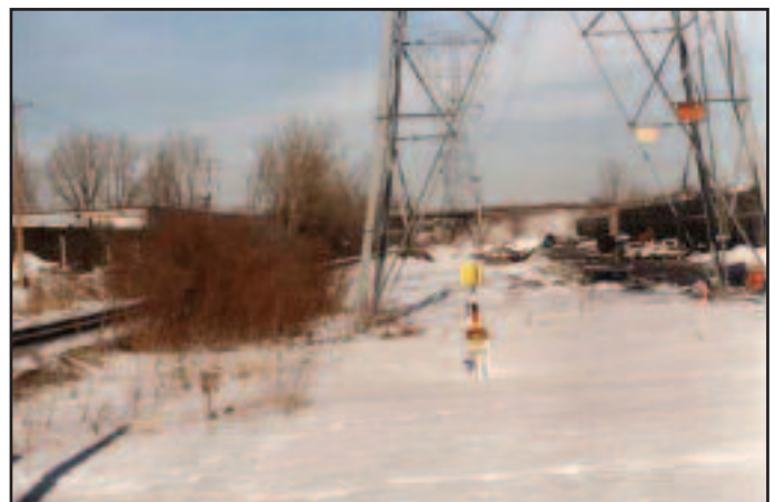
Multiple use of excess land within a 100 foot wide railroad right of way with non-exclusive easements for a pipeline directly under a power line and encroachments for snow storage and parking within both easements. Available space can accommodate other users within the same easement areas.
