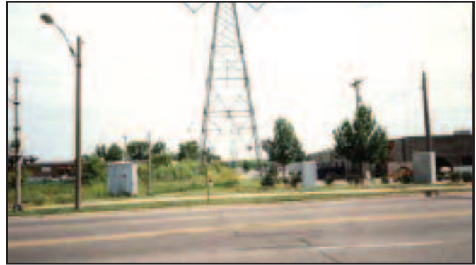
Another multiple use of excess land within a 100 foot wide railroad right of way with non-exclusive easements for a pipeline directly under a power line. Encroachments for parking and (winter) snow storage within both easements from adjacent property. Available space can accommodate other users within the same easement areas.
