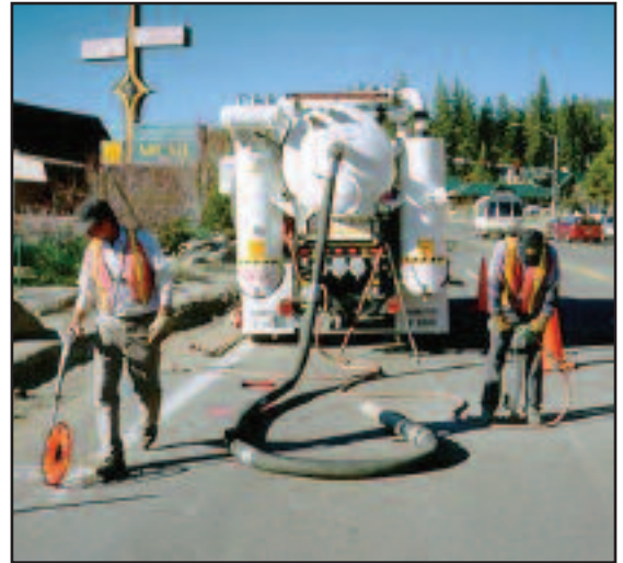
Workers prepare to expose utilities using vacuum excavation
