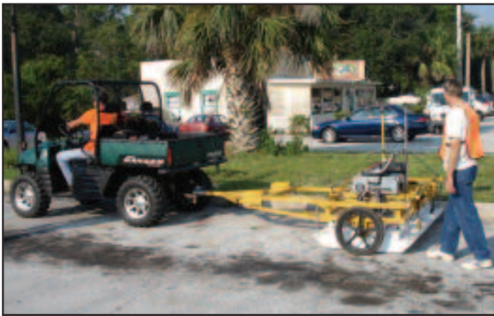
Workers use 3-D underground imaging to designate subsurface utilities.
