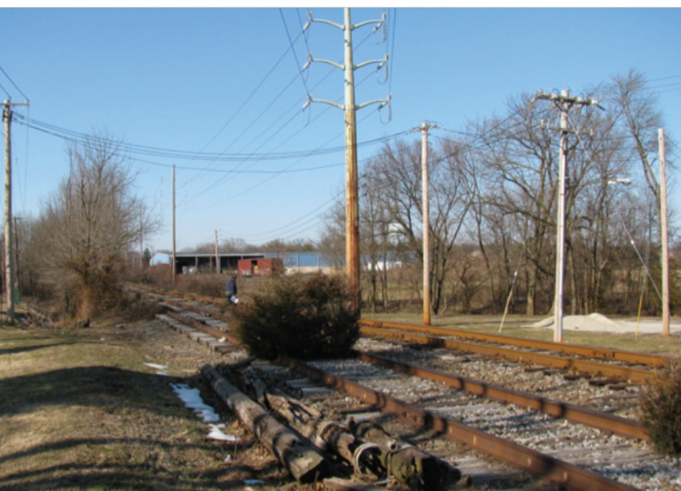
An example of overlapping overhead utility crossings where there is a single license and adjacent public uses.
