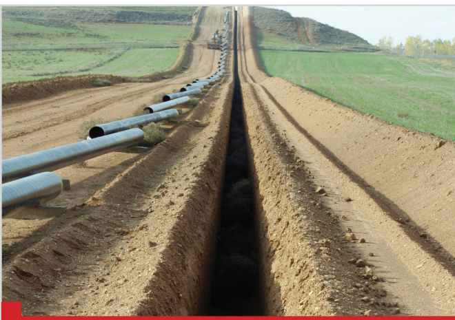
Figure 3: Typical underground pipeline construction methods can be used for Superconductor Electricity Pipelines.
