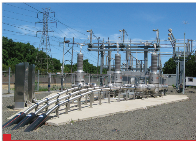
Figure 1: 138 kV AC superconductor power transmission cable operating since April 2008 in Long Island Power Authority's grid.
