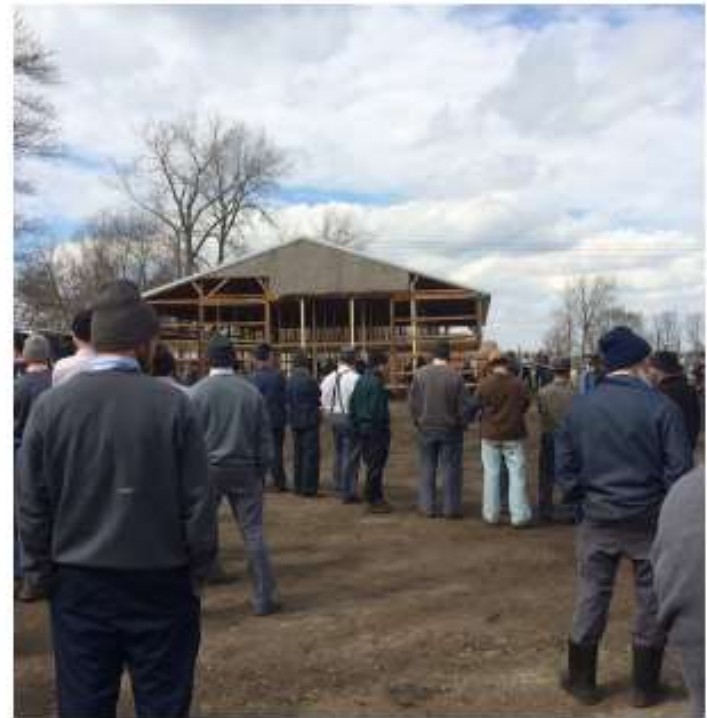
Around 150 Amish men from more than 10 different Amish churches arrive at the barn to assist the landowner in moving the barn to a new foundation out of the way of a new electric transmission line.
