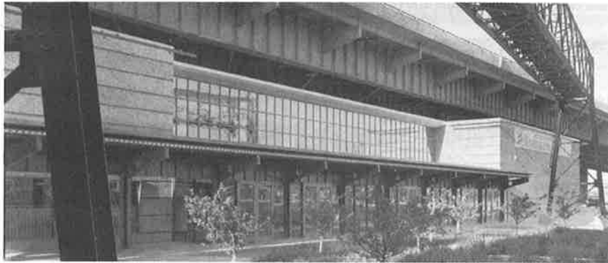
The $6 million, 42,000-square-foot tenplex Union Station Cine seats 2,300 moviegoers. Since it was necessary to go down into the ground, the theater has a steeper slope than normal (all the better to see over the head of the giant who sits in front of you). The trestle in the foreground is one of the original structures on the property, retained to foster the development's railroad atmosphere.
