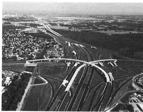
Looking east along I-595 and its four-level $62 million interchange with US 441 (State Road 7). This one interchange has 38 lane miles and 19 of the project's 93 bridges, and occupies a footprint of approximately 300 acres.
