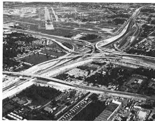
Looking southeast across a major part of the I-595 project nearing completion – the I-595/I-95 four-level interchange and the three-level I-95/S.R. 84 interchange. This $120 million construction contract is DOT's largest ever.
