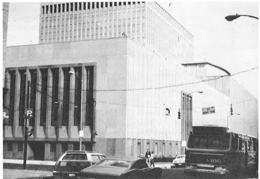
After —The functional replacement of the Central District Police Station (foreground) and Headquarters (background) which was not eligible for replacement.
