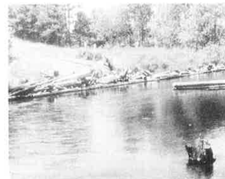
Figure 9. A log jam and wing jam installed to protect a river crossing.
