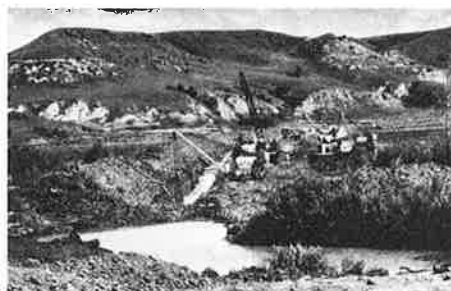
Pipe being weighted down at a stream crossing. (BLM photo)
