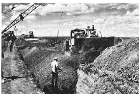
Pictured is a Roscoe-Brown auger backfiller followed by a drag, dozer, and loader. (BLM photo)
