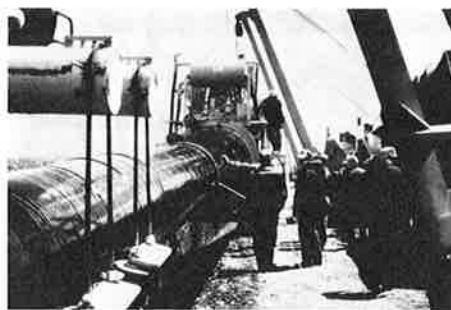
A CRC coating machine cleaning, priming, and covering the pipe with tape. (BLM photo)
