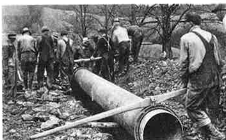
A crew working on Columbia's Seaboard line in 1930 used lifting poles to move pipe into position over the ditch. Each 20-foot section of 20-inch pipe weighed 1,450 pounds.
