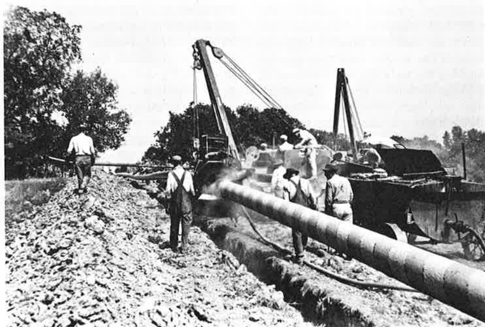
A coating and wrapping machine used in the 1940's put a layer of Cathodic protection between the pipeline and the soil.
