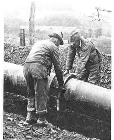
The wrench inspector working on this Columbia line in 1930 made certain all 12 bolts in each coupling were tight.
