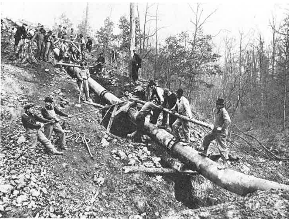
One of the first major transmission arteries of the present Columbia Gas System was this 20-inch pipeline laid in 1916 between Calendenin and Cedarville, W. Va.
