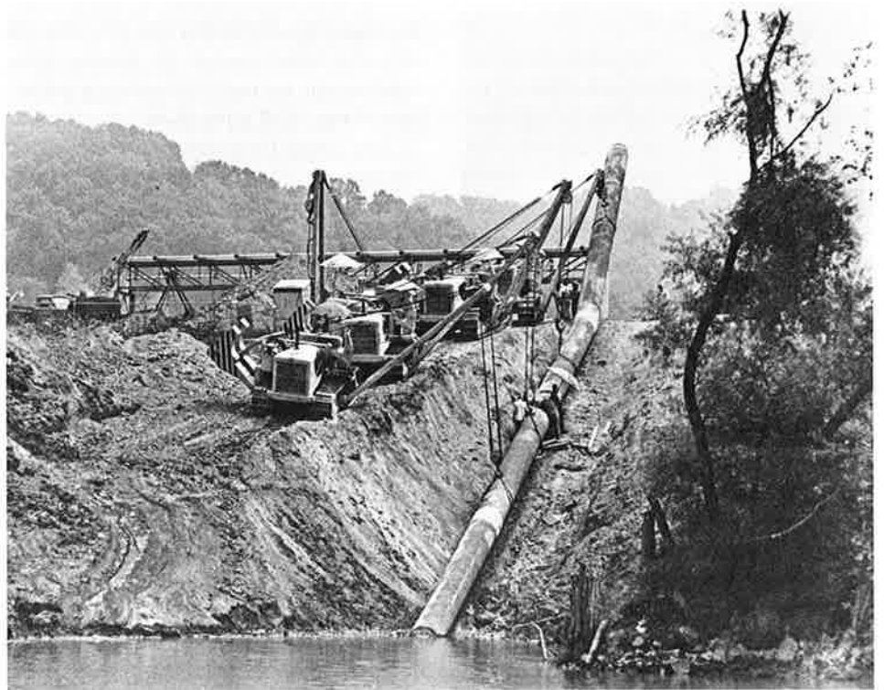
Sideboom tractors have replaced lifting poles for moving the pipeline into the ditch.
