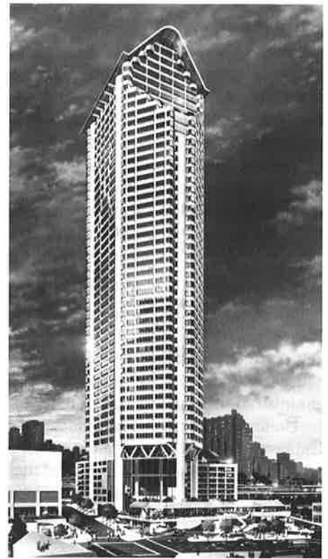
Gateway Tower, Seattle, Washington
