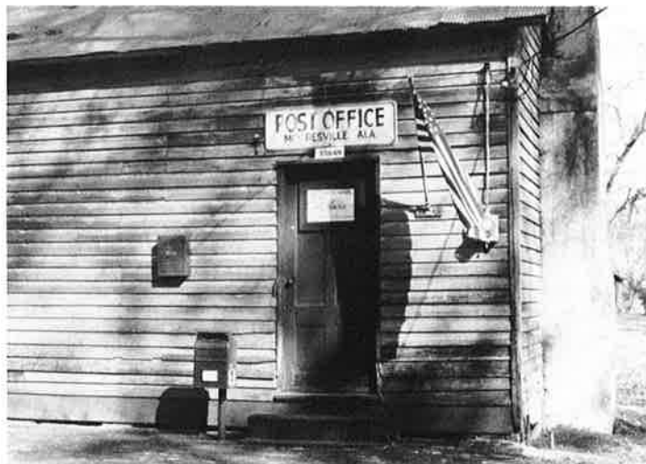
Old historic post office building in the town of Mooresville was within the required right of way.
