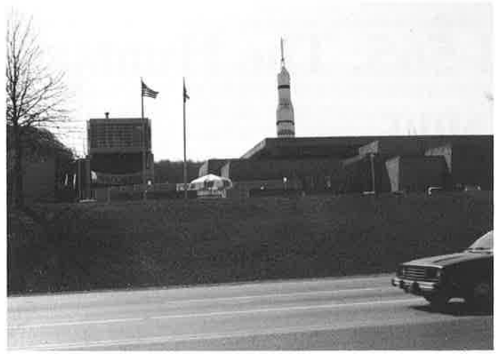
I-565 will run immediately in front of NASA's Space and Rocket Museum.
