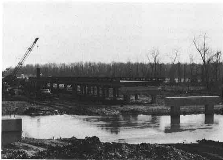
Some bridges in place already where I-565 is superimposed on Alabama Highway 20 were moved over to be used on the frontage roads since they did not meet standards to become part of the interstate.
