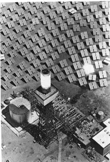
Solar One: The first operating solar conversion unit.
