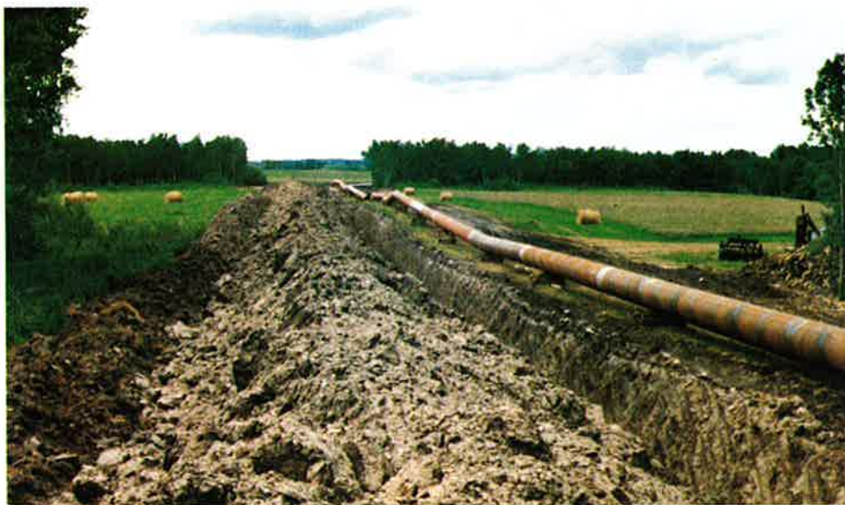
The spoil pile is shown between stockpiled topsoil and the open ditch. Note the narrow width required for this method of topsoil separation. This photo was included in a report titled, "A Preliminary Assessment of the Impact of 1980 Pipeline Construction on Crops and Soils Southeast of Edmonton, Alberta."
