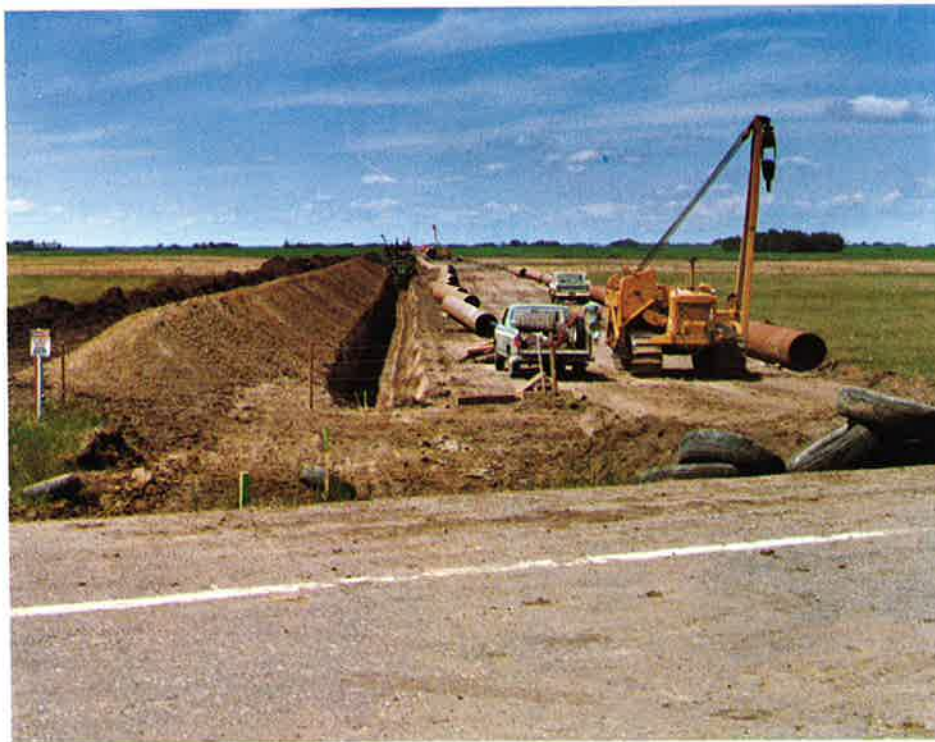
Typical construction layout showing working side, ditch, spoil pile and windrowed topsoil. West of Hwy. 36. This photo was included in a report titled, "A Preliminary Assessment of the Impact of 1980 Pipeline Construction on Crops and Soils Southeast of Edmonton, Alberta."
