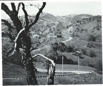
pleasing relationship of road and terrain was achieved by setting maximum sight distances and using combinations of horizontal and vertical curvatures which restrict long distance views of the road segments.
