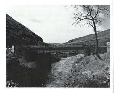
The acceptability of the designs were cleared with the Council of the Confederated Tribes of Warm Springs. The concrete abutments and wing walls were faced with native stone, and the metal bridge rail was painted a bronze color so that the structure would blend in with the surroundings. The site is in an area which has been designated as a Scenic Waterway, which strictly limits construction activity.
