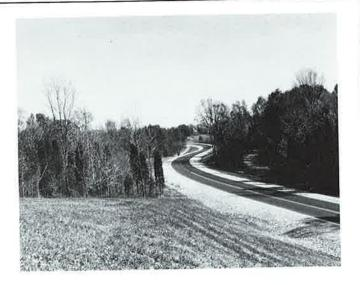
quently scar on the land. This requirement was even more important on this section in Tennessee since the terrain is rolling and hilly. A curvilinear alignment was chosen and a number of rock embankments were incorporated to ensure a minimum requirement for large fills and cuts.
