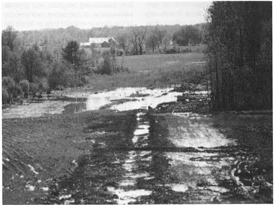
Proper drainage has not been maintained at this site. Note the rutted condition of the right-of-way and the ponded water.
