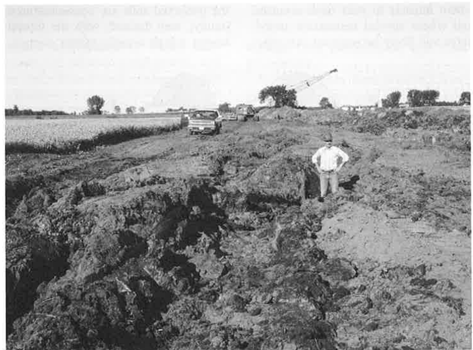
These clay soils were traversed when the right-of-way was excessively wet. As a result, the soil was unable to support the construction equipment without becoming severely rutted. Research has shown that rutting can cause a reduction in a soil's structural stability and other problems which can affect plant growth and development.
