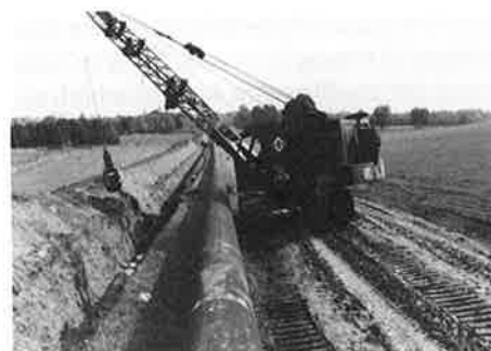
This is an example of pipeline construction under ideal conditions. Topsoil has not been stripped from the work area to protect the subsoil from compaction and erosion.
