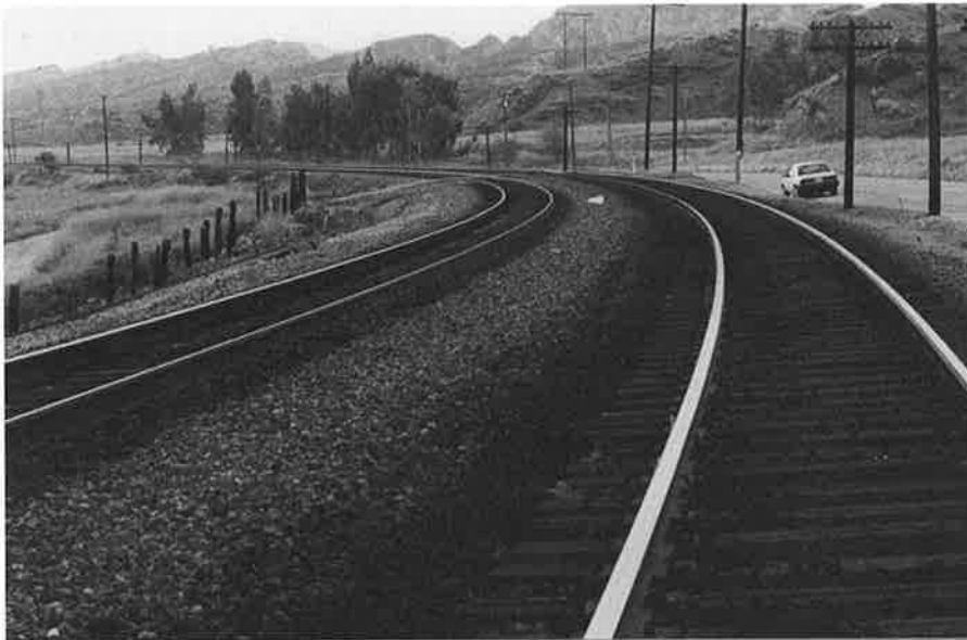
Union Pacific Railroad right of way looking east at approximately crossing of the Inland Feeder. San Timoteo Canyon road is on the right.
