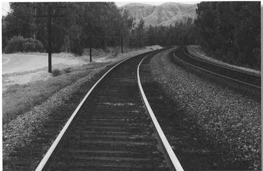
Union Pacific Railroad right of way at approximately Inland Feeder crossing looking west. Inland Feeder will cross from left to right and will be approximately 70 feet below ground surface. San Timoteo Canyon road is on the left.
