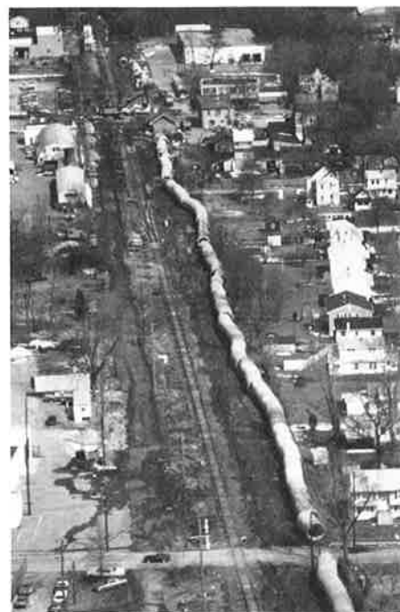
102-inch pipe placed along railroad right of way during construction of aqueduct.
