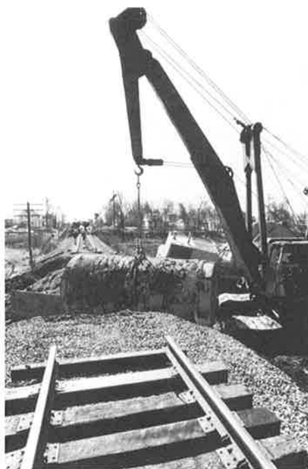
Railroad crossing of 102-inch pipe in Wayne, NJ.
