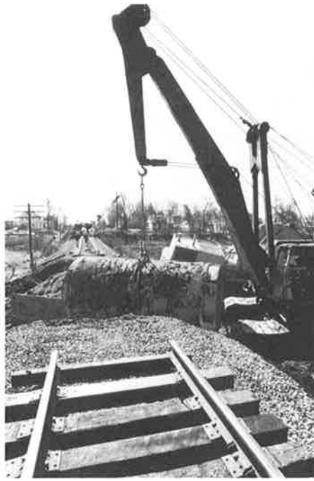
Railroad crossing of 102-inch pipe in Wayne, NJ.
