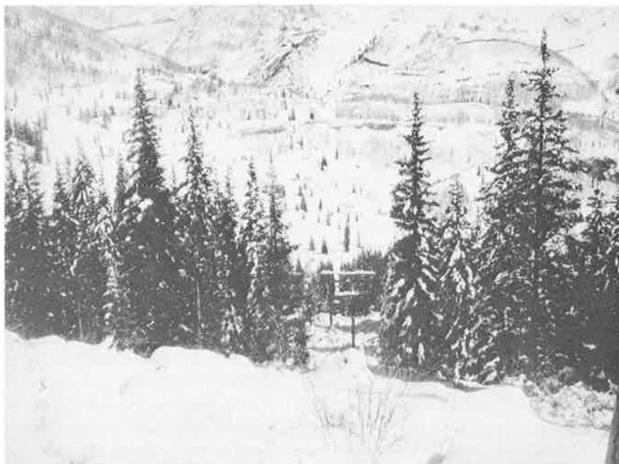
Timber cut to accommodate Pole line Loveland Pass, Colorado
