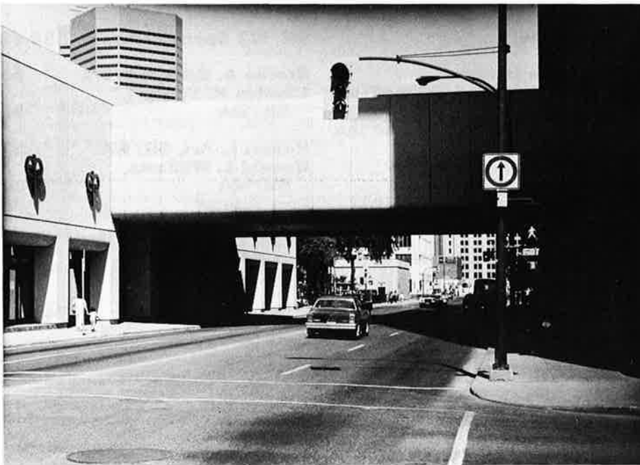
An Example of an Overhead Pedestrian Corridor containing Commercial Sales Space
