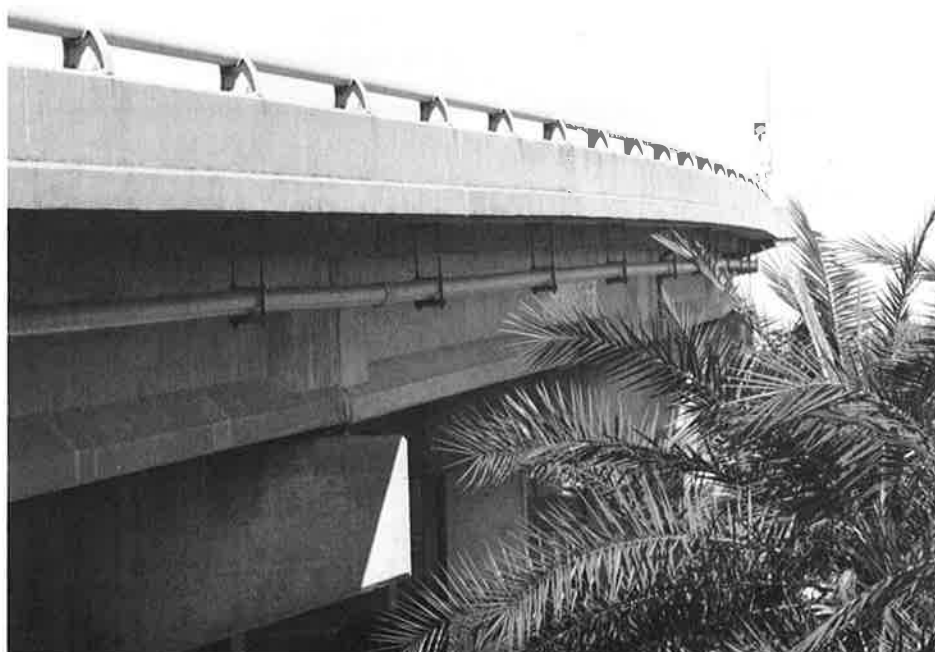
Fort Myers, showing the fiberglass duct housing the fiber optic cable.
