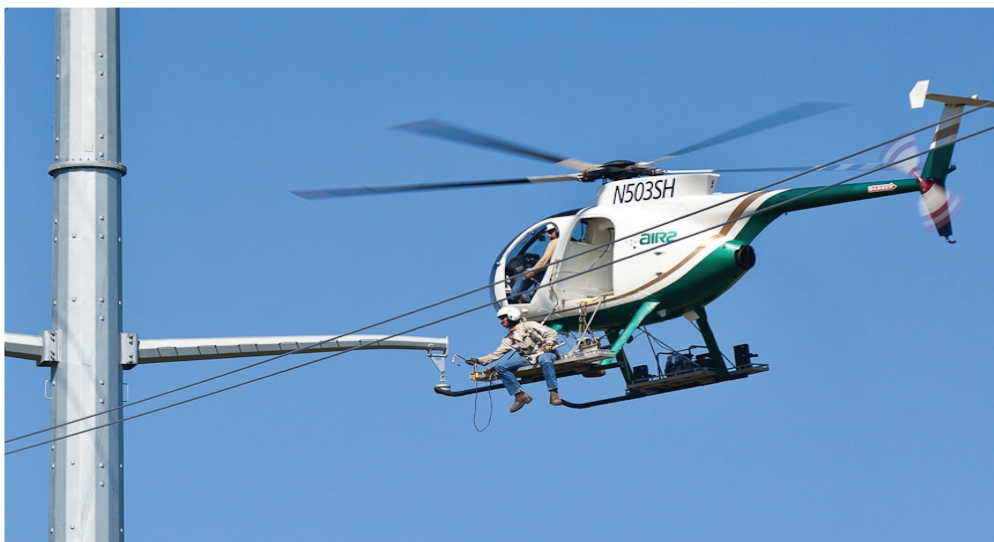
Helicopters were used to string conductor wire for portions of the line, enabling some transmission line work to be performed without placing heavy equipment in sensitive areas, and keeping the project on schedule.
