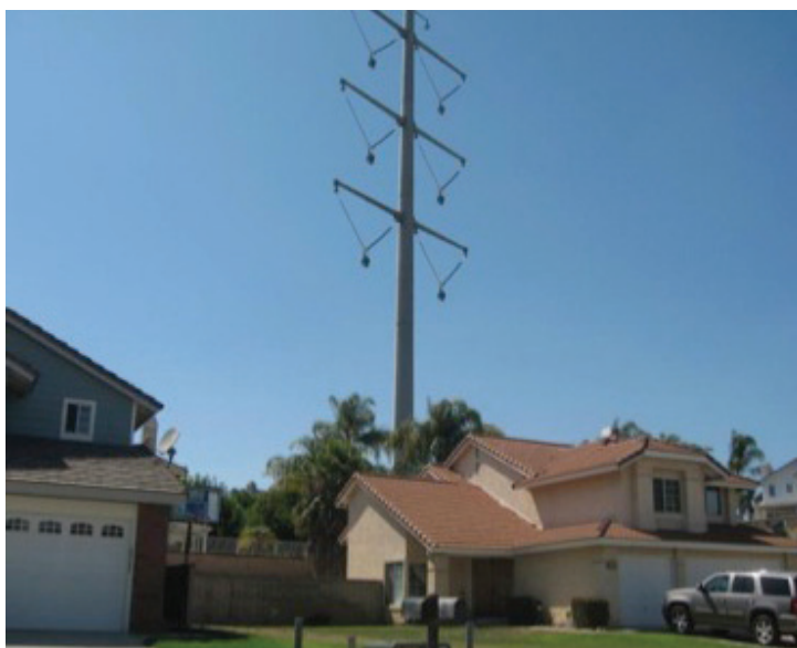
Residents in Chino Hills persuaded the Public Utilities Commission to suspend construction and underground a 3.5 mile segment, causing $220 million in incremental legal and construction costs.
