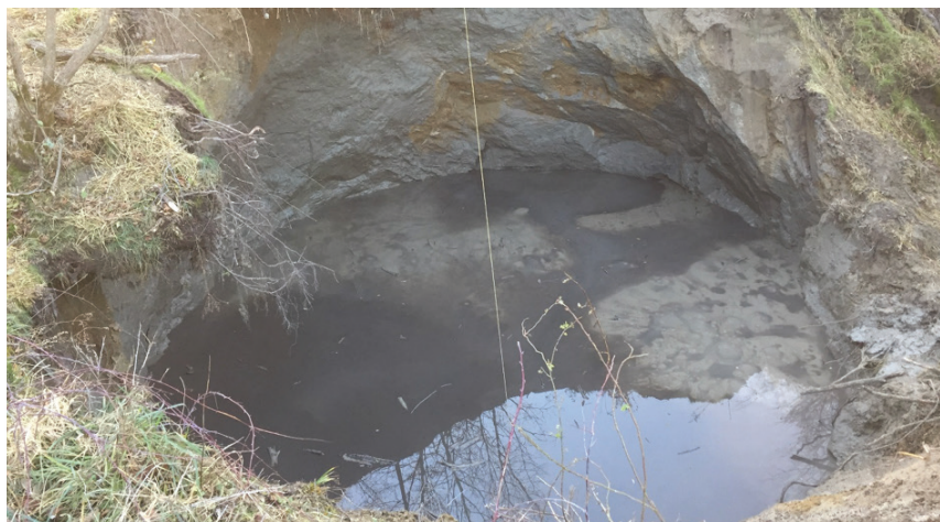
Post construction sink hole discovered during right of way survey.
