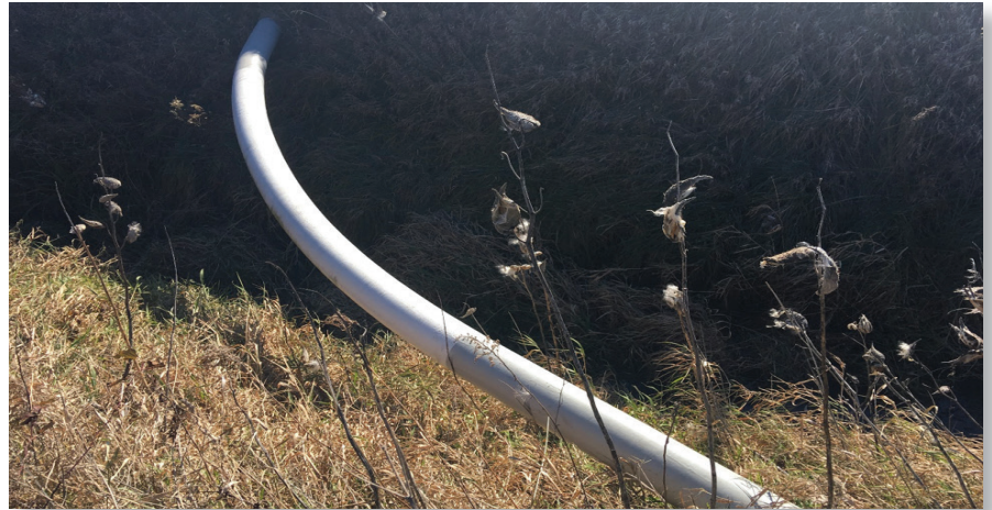
Fusion bonded epoxy coating inspection during right of way patrol.
