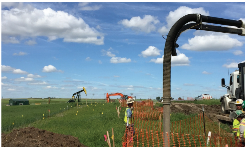
Watch and protect activities during foreign line crossings of existing utilities with 811 best practices in effect.
