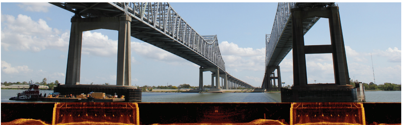
For submerged bridge inspections where diving conditions are hazardous, Fenstermaker has proven the effectiveness of underwater acoustic imaging.
